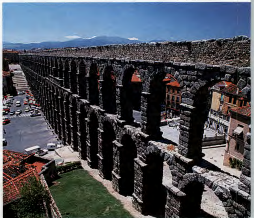
Figure 9 ▶ This Spanish aqueduct was built almost two thousand years ago by the Romans.
