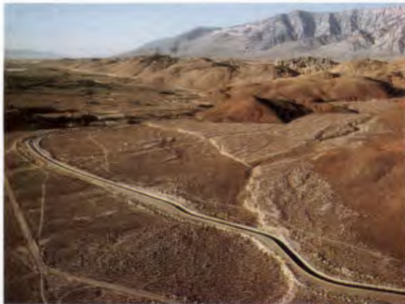
Figure 10 ▶ This canal carries water more than 300 km across mountains and deserts to supply drinking water to Los Angeles, California.
